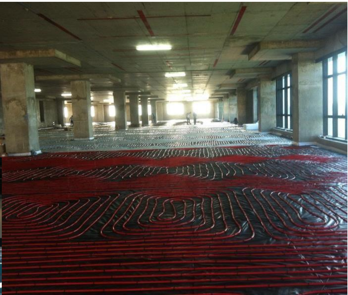
Floor Cooling – Installed in 2014
